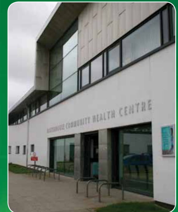
Easterhouse Health Centre
